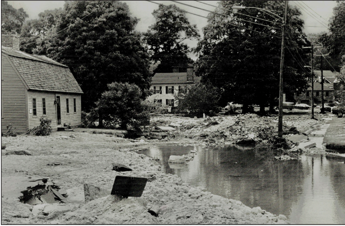
North Main Street Suffered Major Damages
