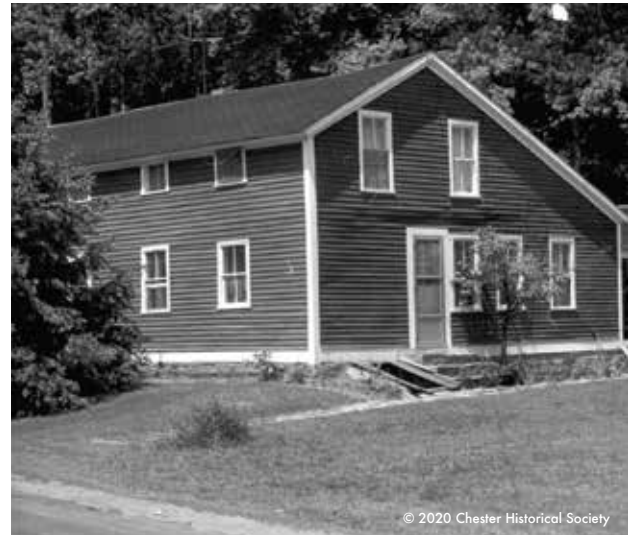
The Dunk House before its 1976 restoration.
