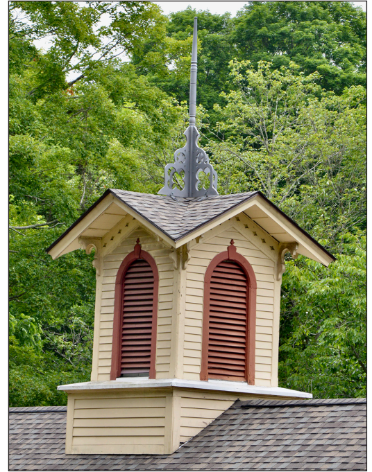
Following the installation of new roof shingles and gutters at the museum, member Art Christianson crafted a handsome spire to top the cupola, replicating the historic one that fell a few years ago.
